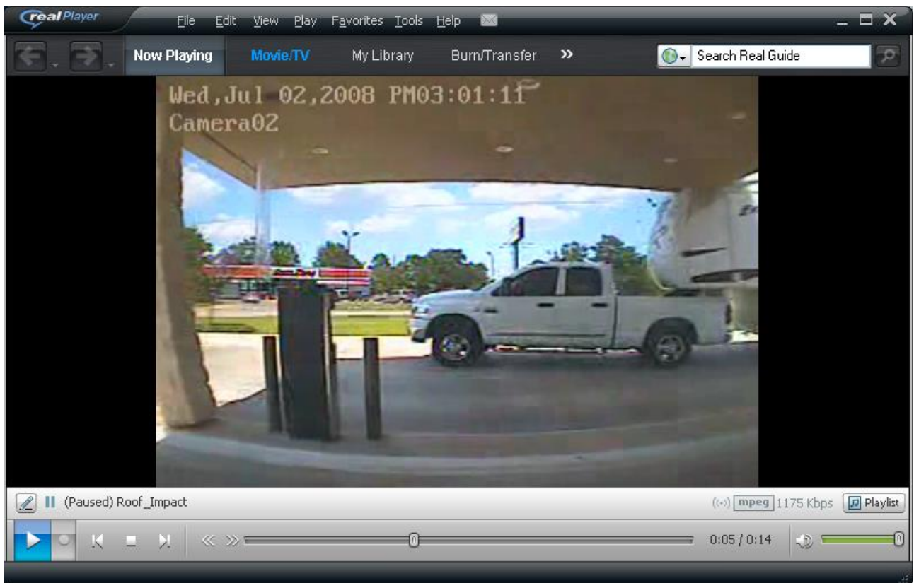
Figure 10 – The Roof Collapsed because the Columns Fell, Not because the Trailer Hit the Roof
